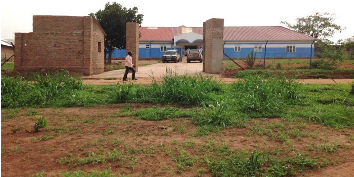
A facility in Kibaale completed and furnished with HBVP revenues
