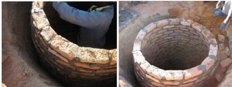
A pit lining from the Blair Ventilated Improved Pit (bVIP) latrine in Zimbabwe. (Photo: Peter Morgan 2011)
