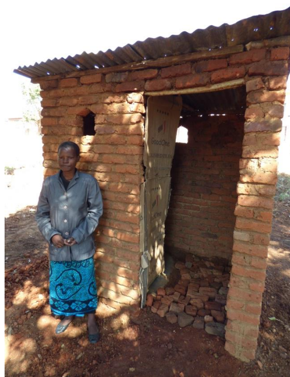
A homeowner stands in front of her newly constructed transitional latrine.
