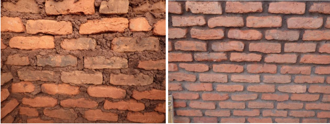
Different techniques are used to mortar walls. The left photograph shows a wall with unfinished mortar and the right shows a wall with finished mortar.
